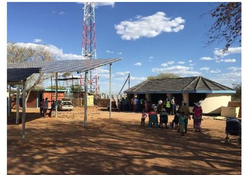
One of the more interesting aspects of this project is the direct comparison of the performance of the three types of panels (1 kW of monocrystalline silicon panels, 1 kW of polycrystalline panels, and 1 kW of amorphous silicon panels) under the energetic and harsh Botswana sunlight. UB researchers will be able to monitor their performances over the short and long term to determine which would be best for the high irradiation conditions here.
